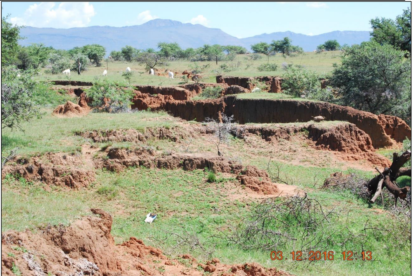
The surrounding floodplains and catchment areas are highly degraded due to overgrazing, resulting in erosion and donga formation.
